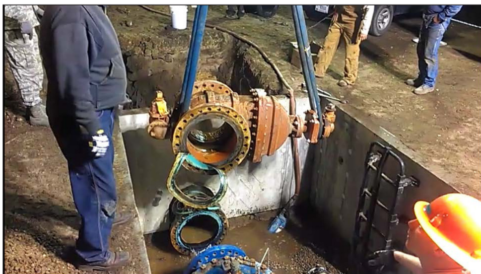
Figure 6: Repairs to a Potable-Water Pipe on Vandenberg Air Force Base
