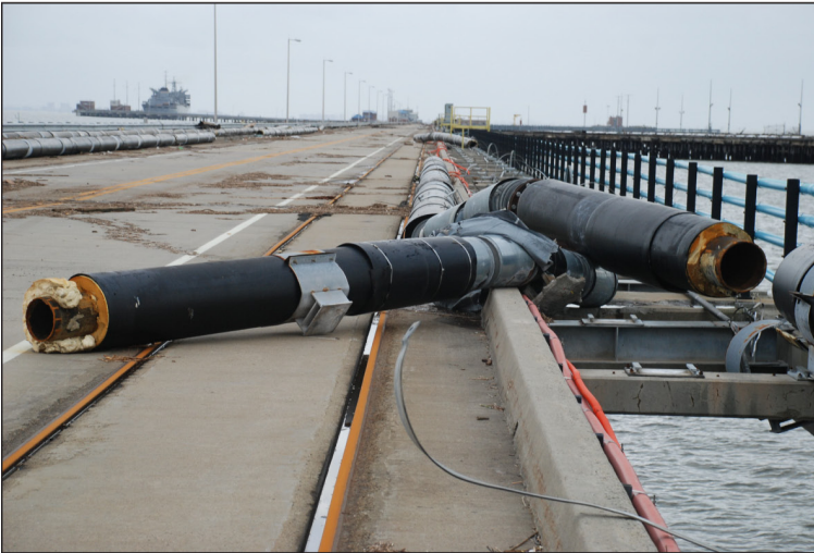
Destroyed by Hurricane Sandy
