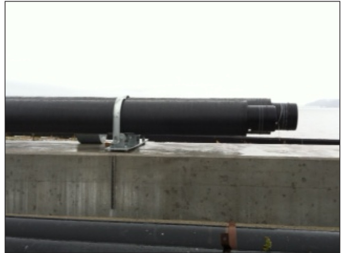
New, strengthened water lines being installed
